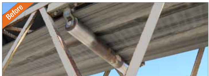
This Belt was Eating into Brackets and Ripping
