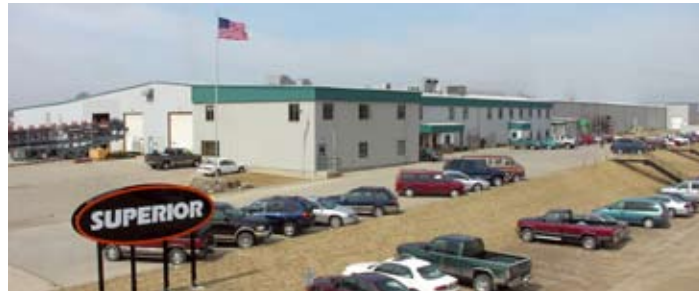
EQUIPMENT DIVISION | MORRIS, MINNESOTA
