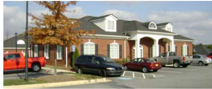
FESCO SYSTEMS DIVISION | NORCROSS, GEORGIA
