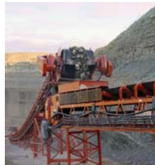
OVERLAND CONVEYOR SYSTEMS
